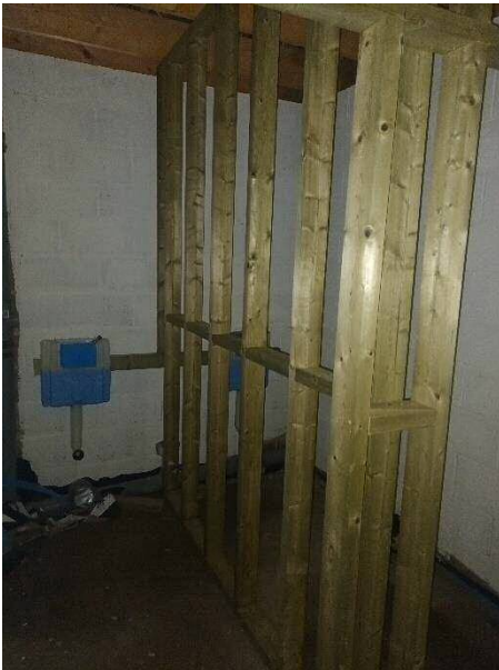
Toilet area going in
