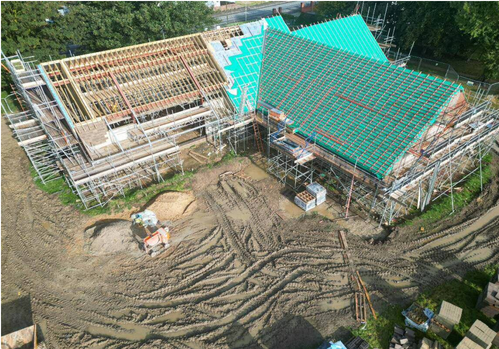
Roof starting to take shape
