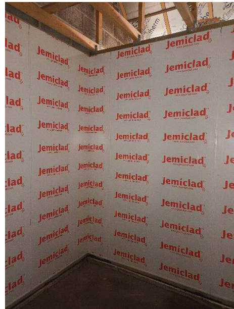
Rooms taking shape
