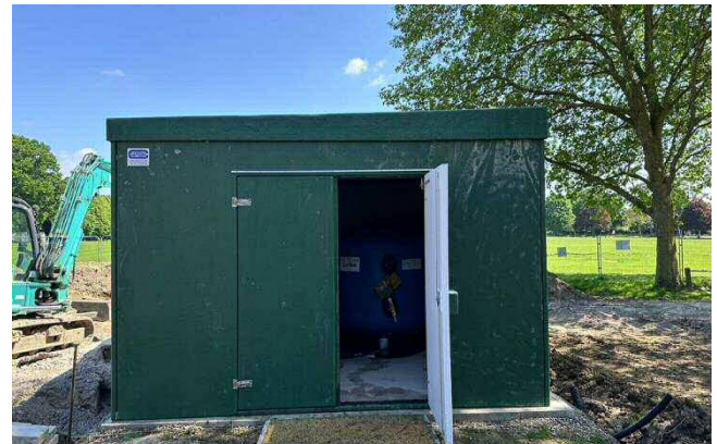
Plant room built
