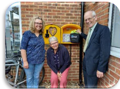
Grant for Defib Machine installed at Didcot Baptist Church
