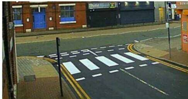
: Example of a non-prescribed zebra crossing at one of the trial sites (from
