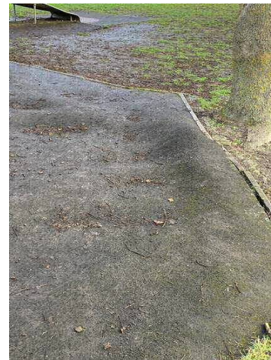
Tree roots lifting the safety surface.
